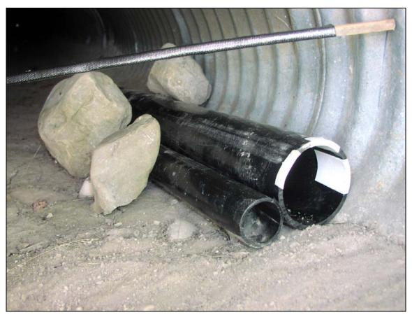
Pipes placed in culverts to provide cover for small mammal movement (Photo: Tony Clevenger).
