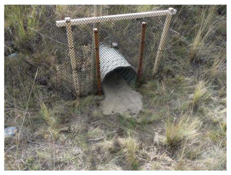
Culvert retrofitted as badger culvert with fencing, east of Cranbrook, BC (Photo: Trevor Kinley).
